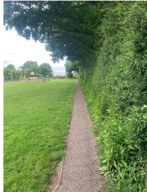
Photograph 10: Footway at Recreation Ground
